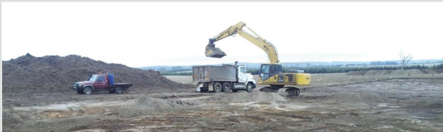
Site establishment works
