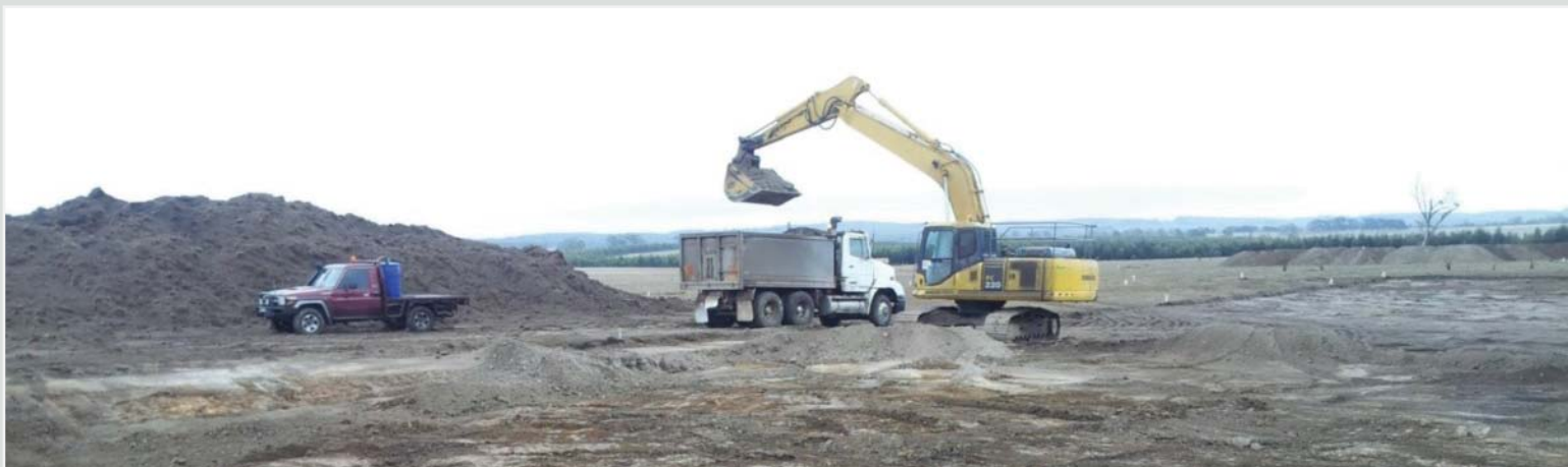
Site establishment works
